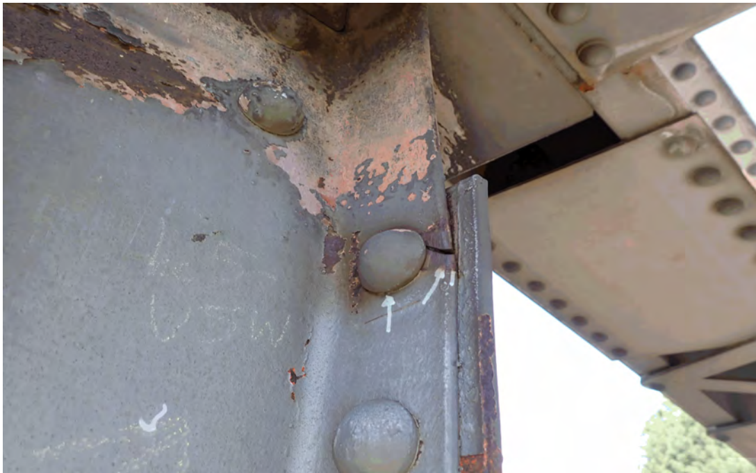
(CS 3) Crack in the northeast flange of L5W-U5W at U5W.
