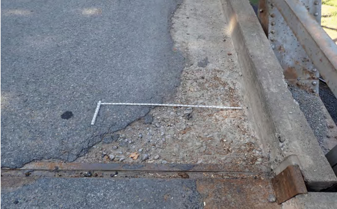
(CS 3) Spalling in the top of the deck at the north end of span 7 looking south.
