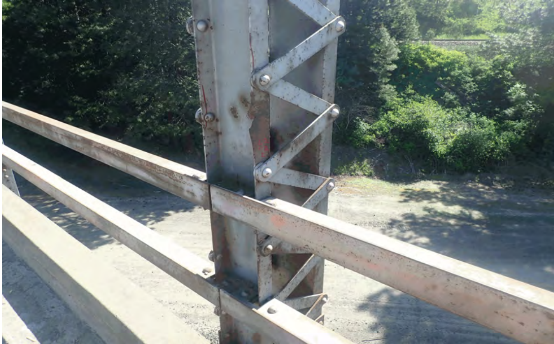
Impact damage to L2E-U2E looking north.
