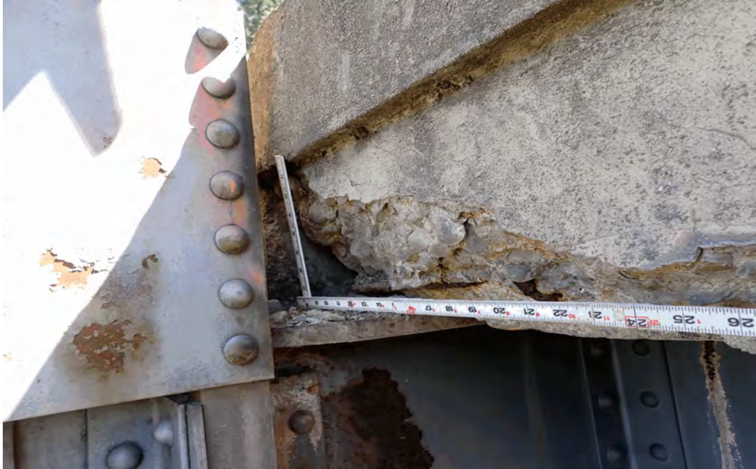
(CS 3) Spall in the west edge of the deck at floorbeam 6 looking north.
