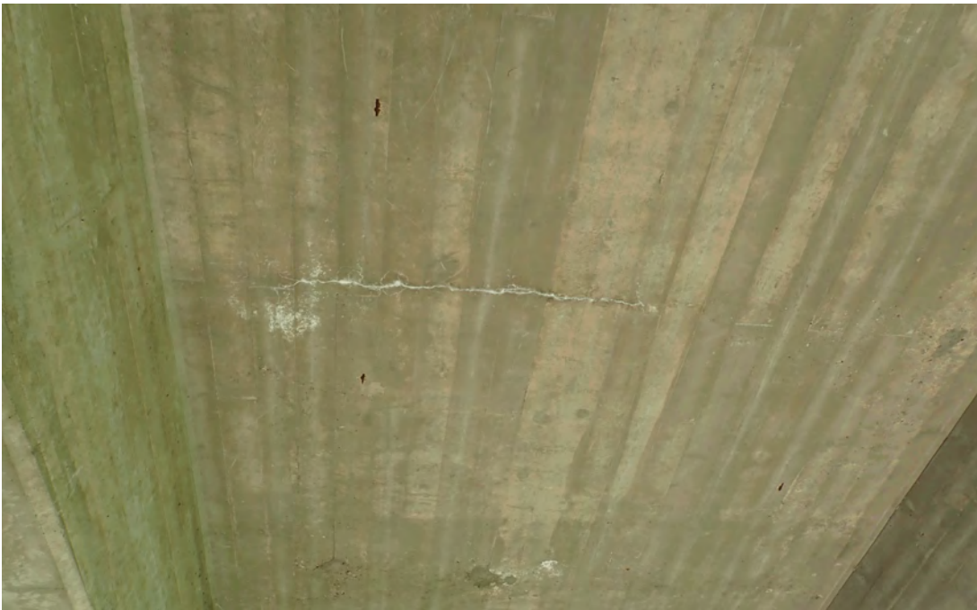
Typical cracking with efflorescence in the underside of the deck.
