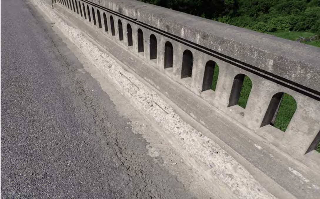
Typical spalling of the curbs in the approach spans.
