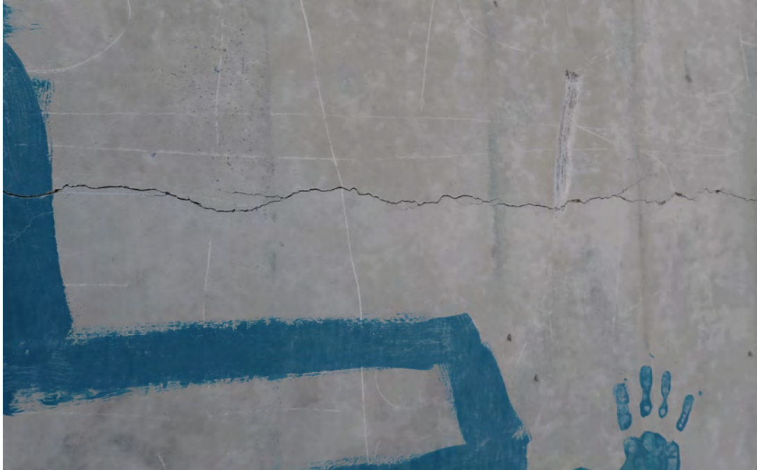
Typical cracking in the pier walls.
