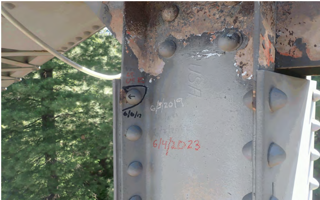
(CS 3) Crack in L5E-U5E at U5E.
