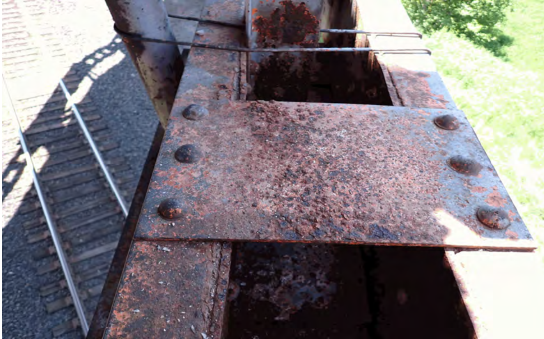
(CS 3) Typical pitting in L3E-L4E looking south.
