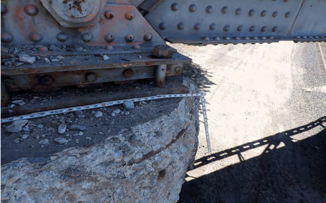
(CS 3) Spalling and deterioration of the cap at pier 7.
