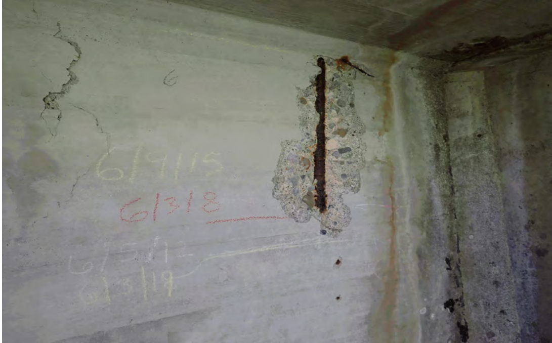
Spall in the west exterior girder at the south abutment looking east.
