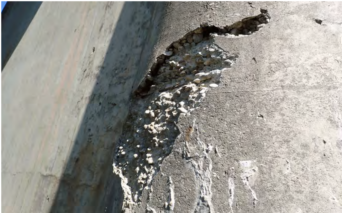
(CS 3) Spall in the south face of column 2 at pier 6 looking northwest.
