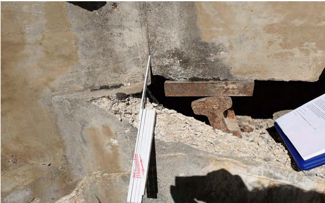
(CS 3) Spalling of the southeast bearing at the south abutment looking west.
