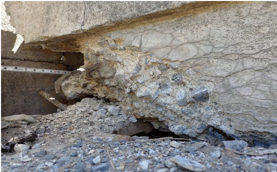
(CS 3) Spall in the northwest corner at floorbeam 7 looking northeast.
