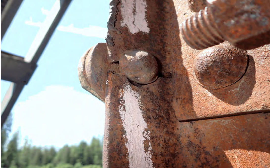
(CS 3) Crack in the northeast flange of L5W-U5W at the lower sway brace connection.
