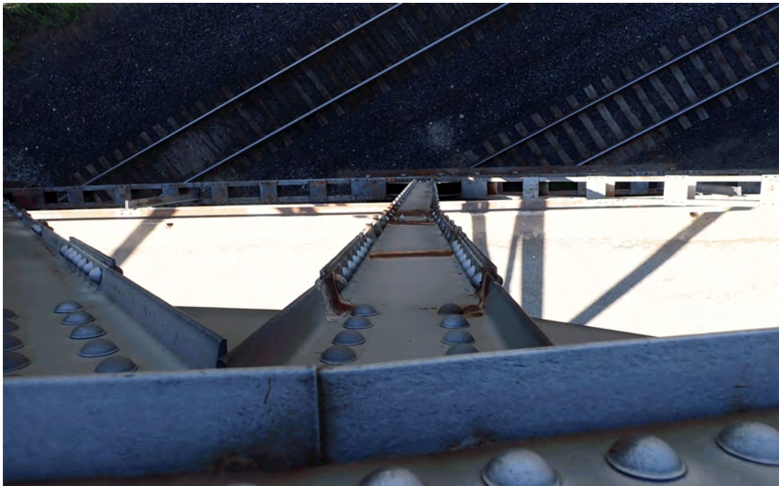
(CS 3) Distortion in L5W-U5W.
