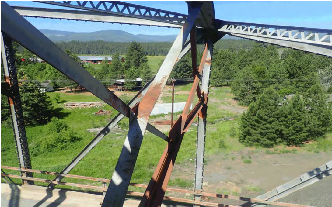
(CS 3) Impact damage to U5W-U5E sway brace looking west.
