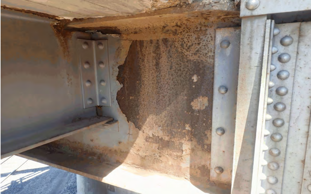
Typical corrosion at the floorbeam ends.
