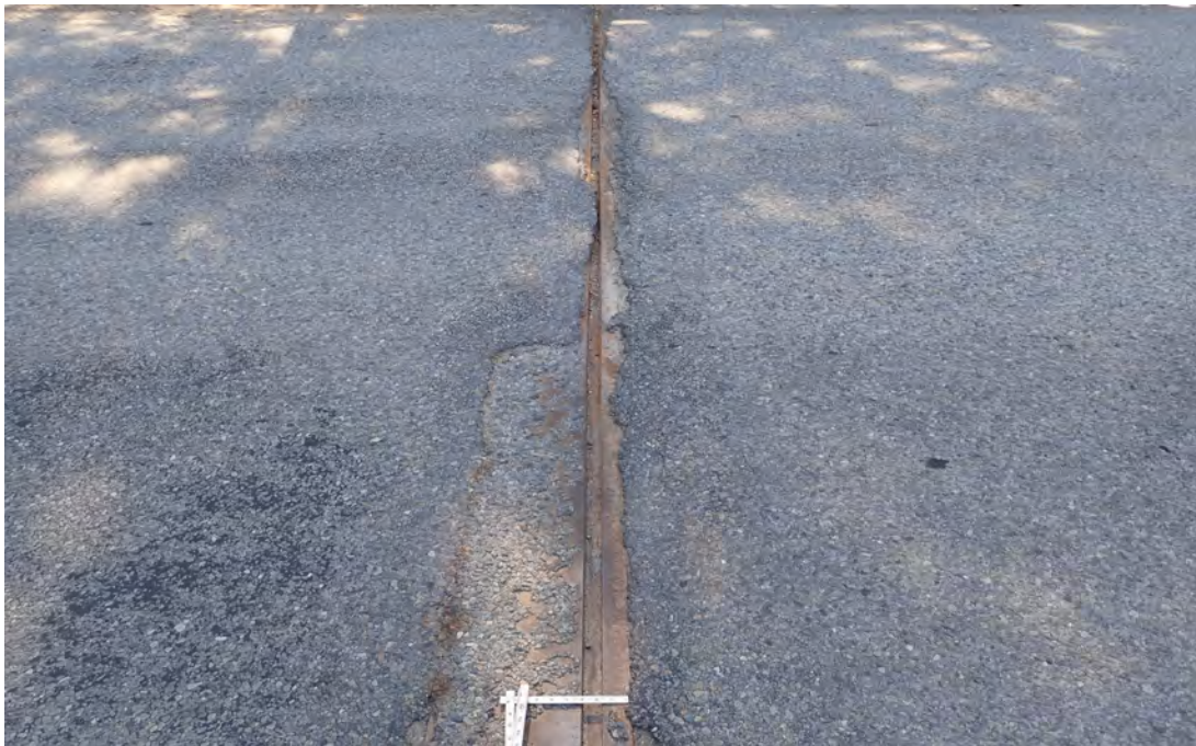
Joint over the north abutment looking east.
