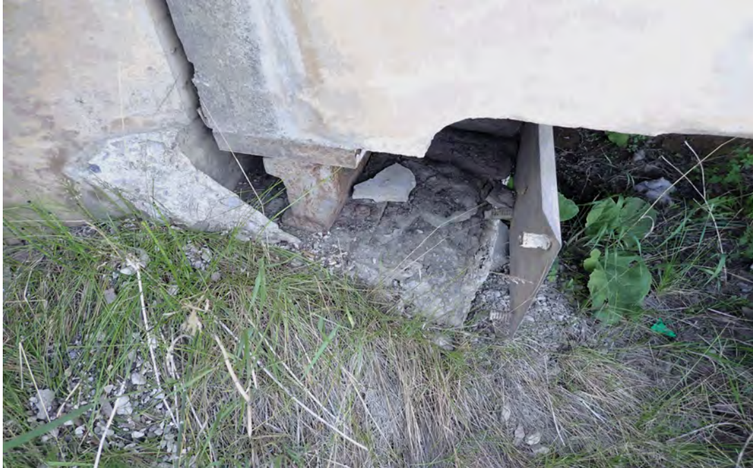
(CS 3) Spalling at the northwest bearing at the north abutment looking east.
