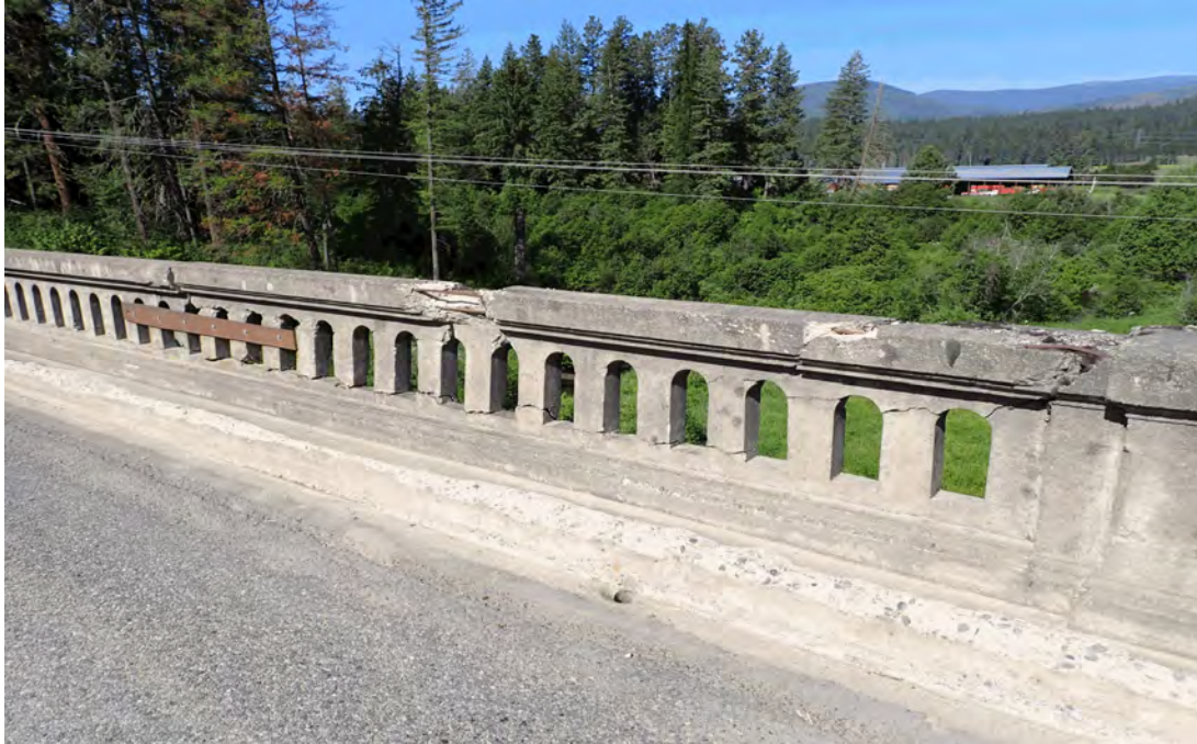
(CS 3/4) Broken bridge rail on the west side of span 4 looking southwest.
