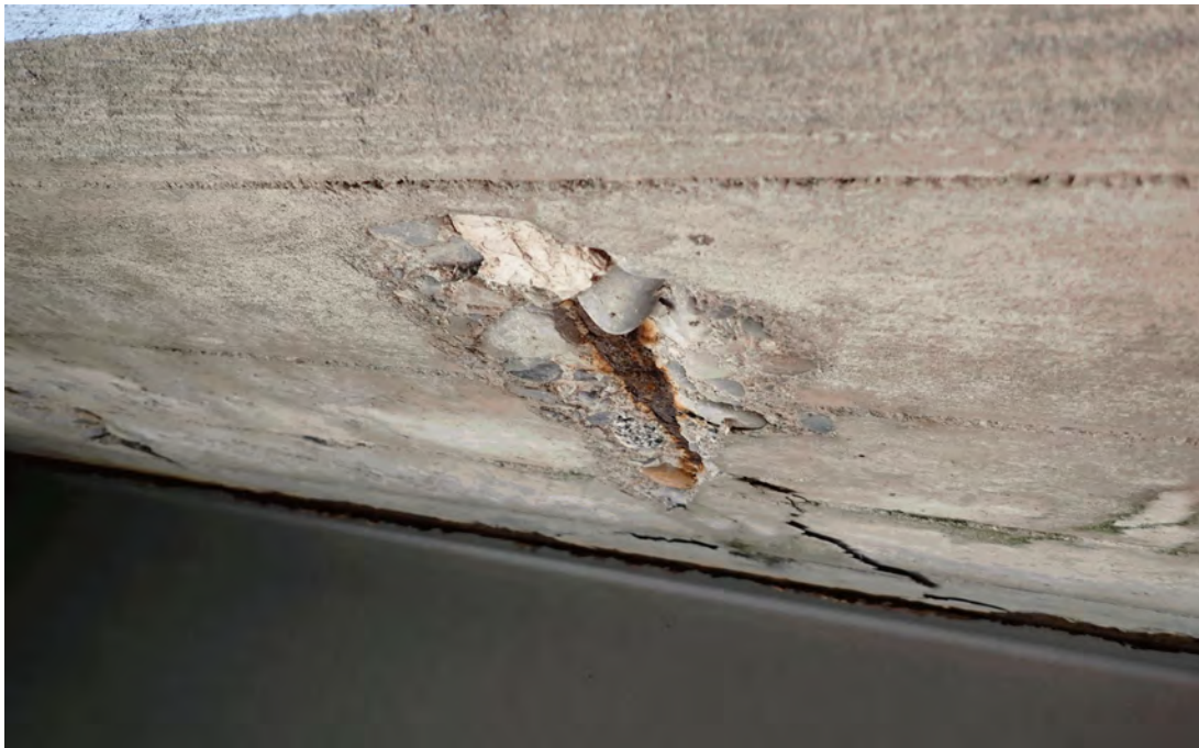
(CS 3) Typical spall in the underside of the deck.
