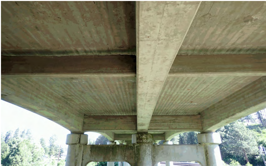
Typical underside condition of the approach spans.
