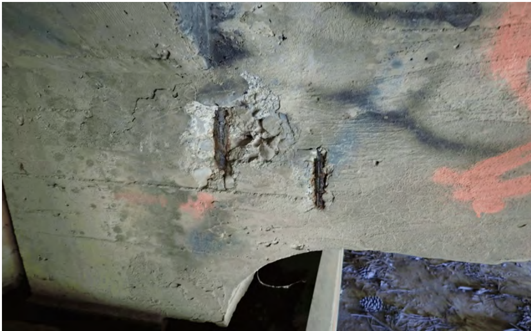
(CS 3) Spalling with exposed and corroding rebar in the center girder at the north abutment looking east.
