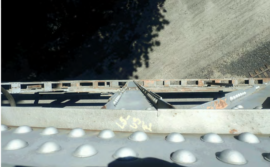
(CS 3) Distortion in L5E-U5E.
