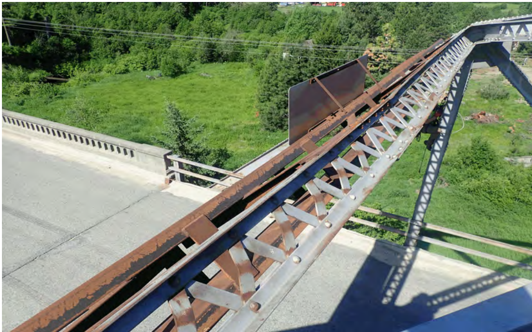
Impact damage and distortion to the south portal looking southwest.
