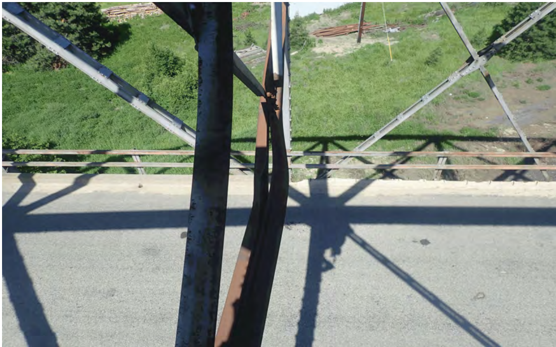
(CS 3) Typical impact damage to sway bracing.
