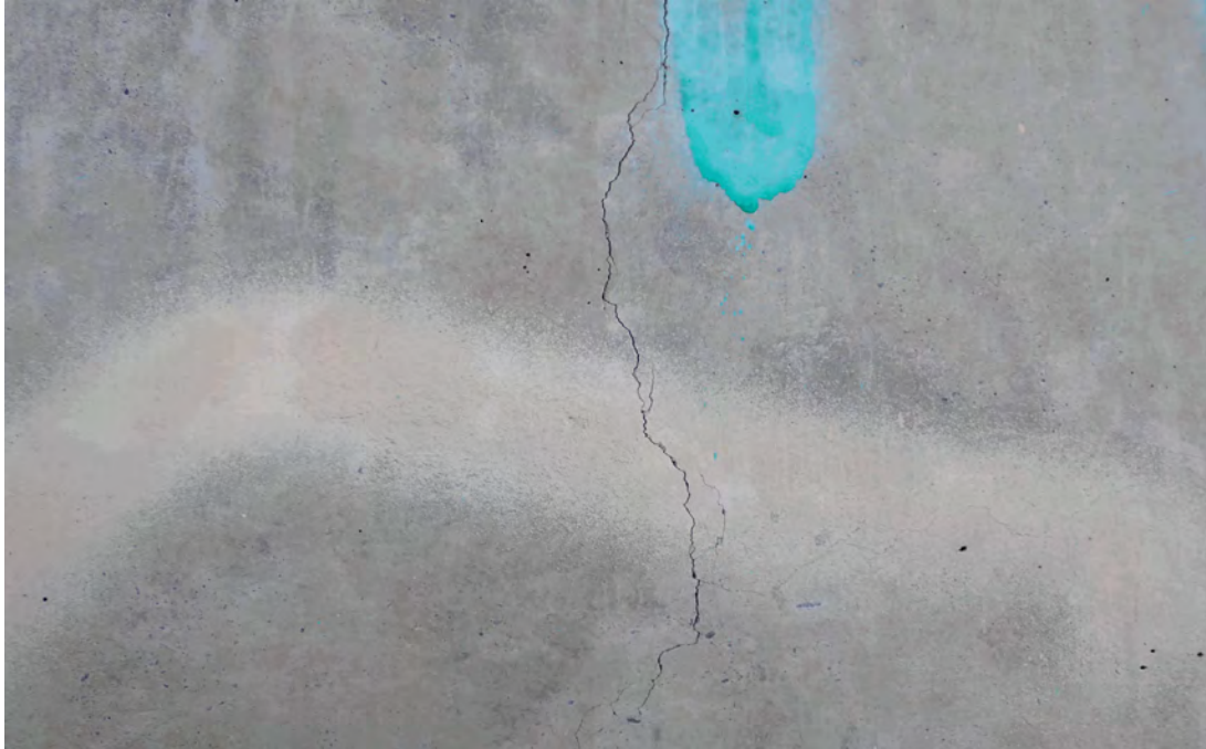
Typical cracking in the approach span girders.
