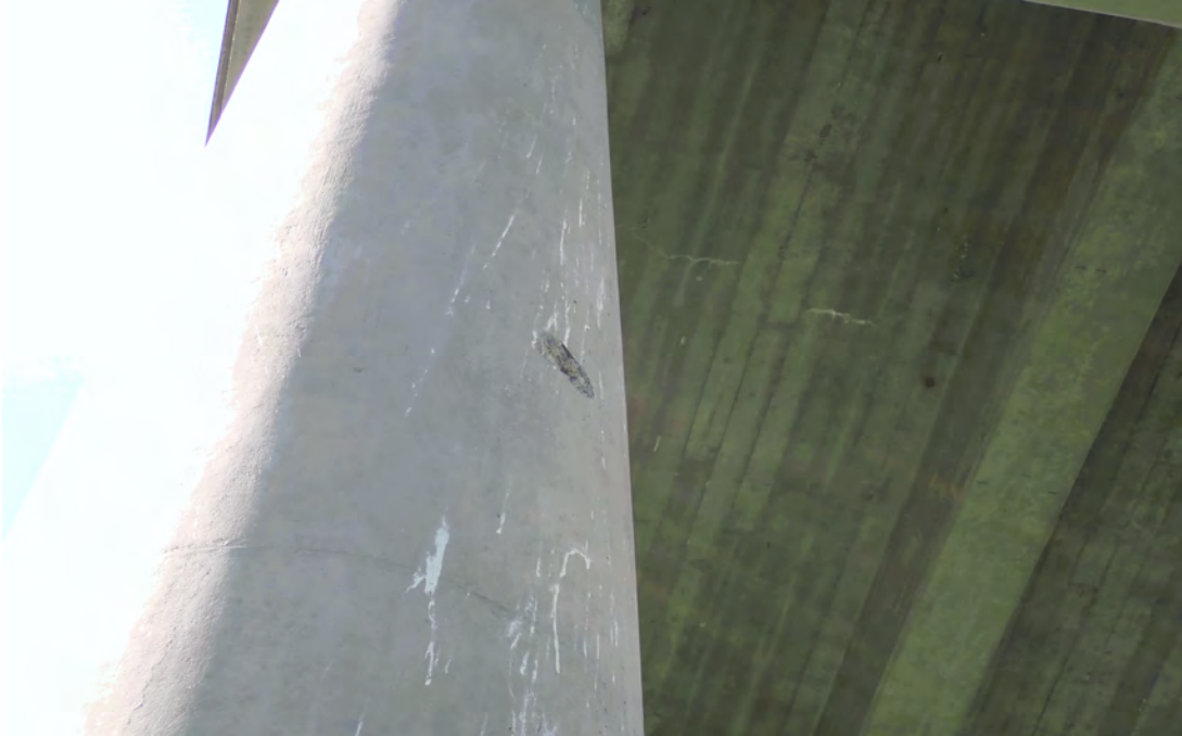
(CS 3) Spall in column 3 at pier 4 looking south.
