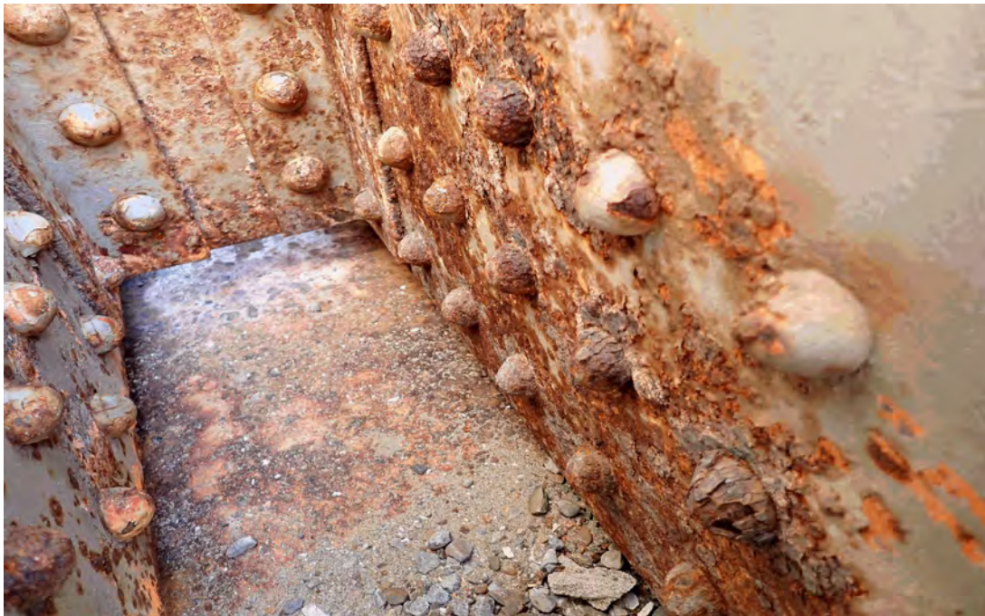
Typical corrosion of the rivet heads on the bottom chords.
