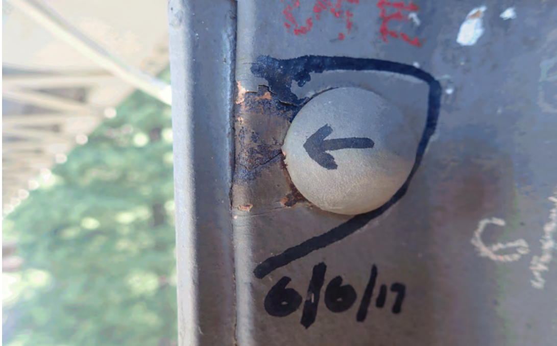
(CS 3) Crack in L5E-U5E at U5E.
