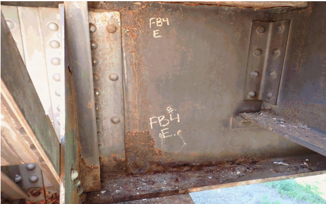
(CS 3) Typical areas of corrosion with loss of section on the floorbeams.
