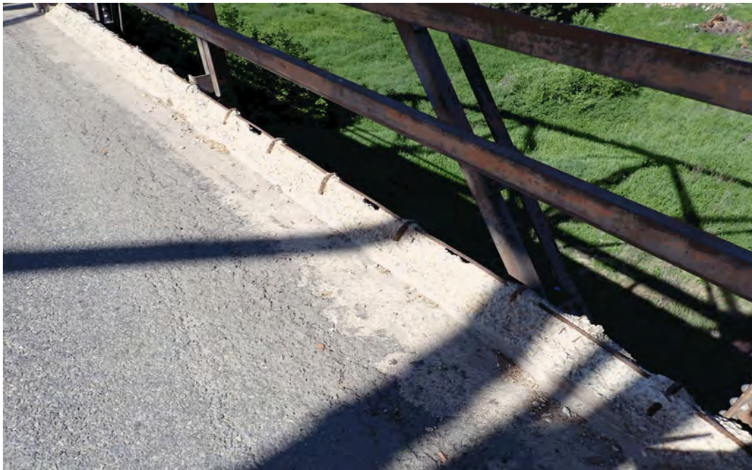
Typical spalling of the curb in the truss span.
