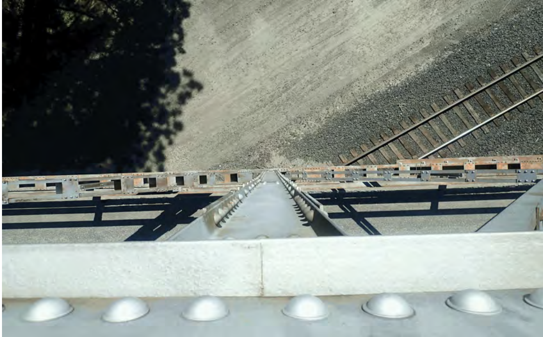
Out of plane bending in L4E-U4E.
