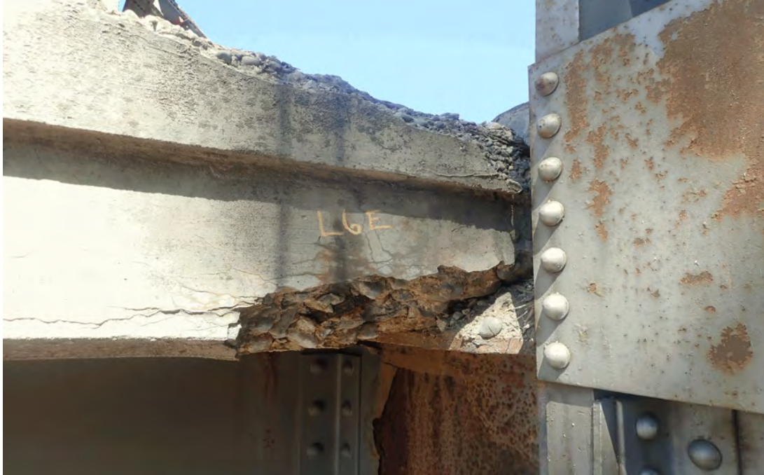
Spall in the east edge of the deck on the south side of floorbeam 6 looking northwest.
