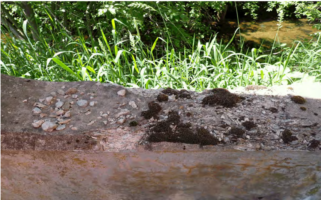
(CS 3) Typical spalling in the top of the lower pier 3 wall looking south.
